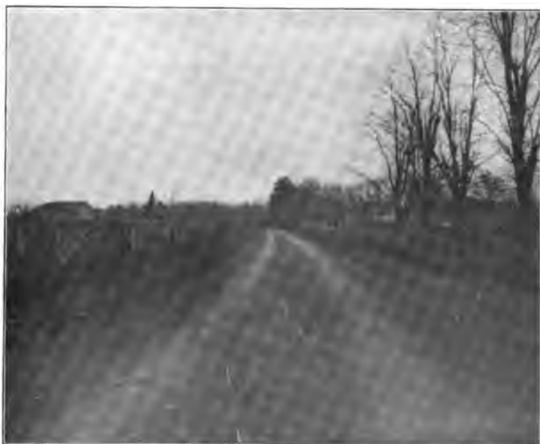
Looking toward Crosswicks on Bordentown and Crosswicks turnpike, Burlington Co., after completion.
